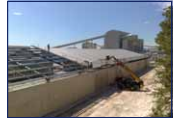
▲ The building is nearly water tight.
