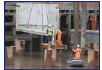
▲ Installing the first PCC segment for the Pintol foundation
