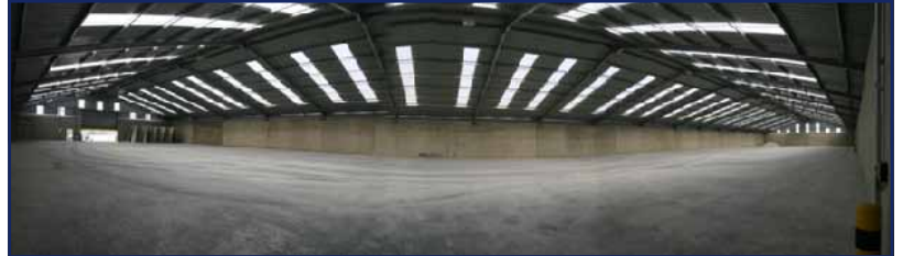
▲ Interesting inside shot of the completed Bulk Store - thanks to clever photography, curved walls and ceilings were all in a days work!
