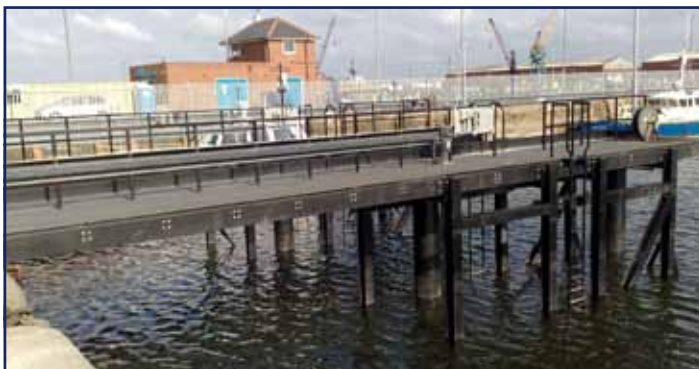
▲ The finger piers of the boat hoist
